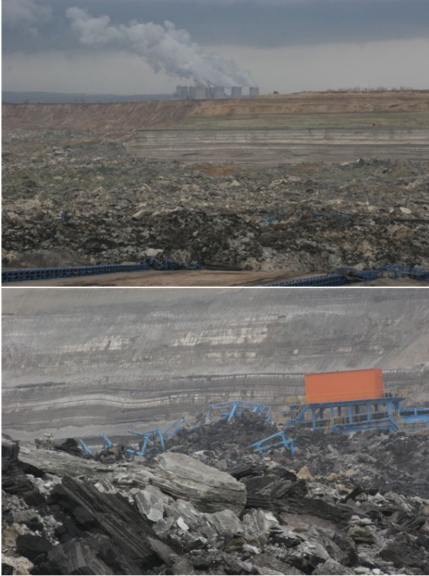
Figure 1: Overview of a real-world accident where a complete daylight coal mining site has collapsed. Several people have been killed and many objects have been buried.
